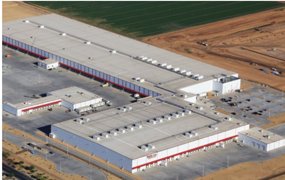
■ To ensure this 902,000-square-foot distribution center was completed in just 48 weeks, ESI Group allowed bidding and construction to proceed without completed design documents.
